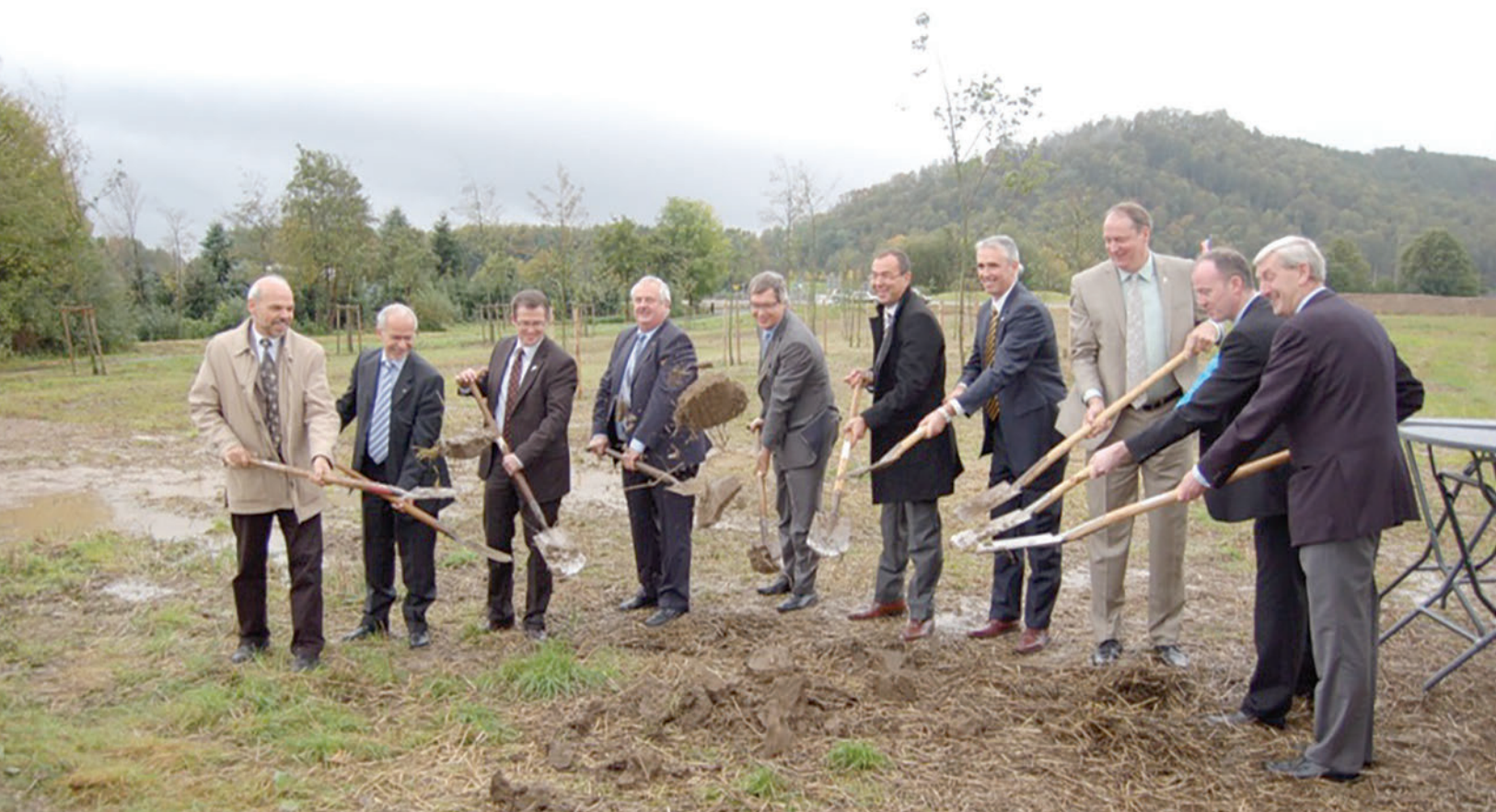
► The ground-breaking ceremony for the EMEA Distribution Centre, which took place on October 19, 2010.
