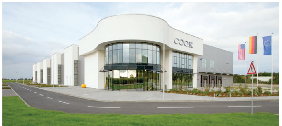
▲ The construction for the EMEA Distribution Centre was completed on August 19, 2011.
